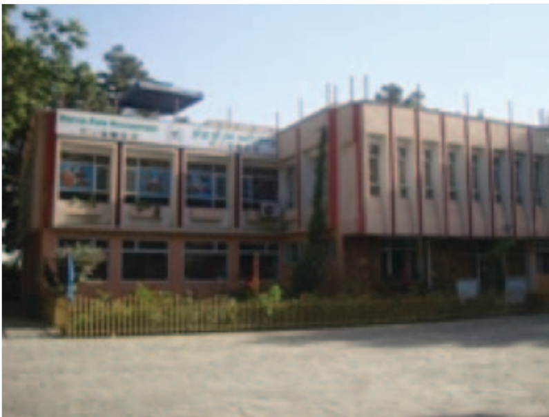
The main building of zoo have a restaurant made by ECO project and now started service of food for visitors by name of (Marco Polo Restaurant) which the zoo had a restaurant by this name 46 years ago.
