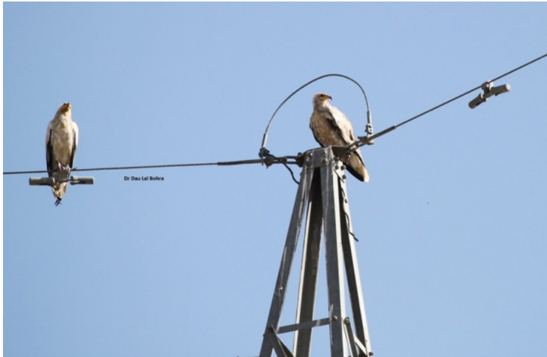
Egyptian Vultures on pylon.
