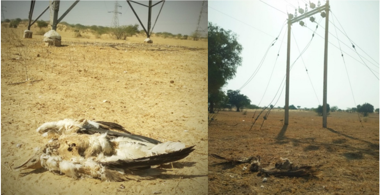
Egyptian Vulture mortality by power lines.
