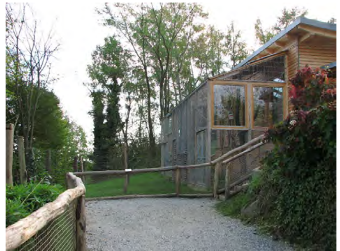
Visitor area: The netted exhibit has glass windows in the upper part next to the visitor area and a double door for bringing in trunks and branches. Steps take the visitors to the upper viewing area ©Monika Fiby, 2014
