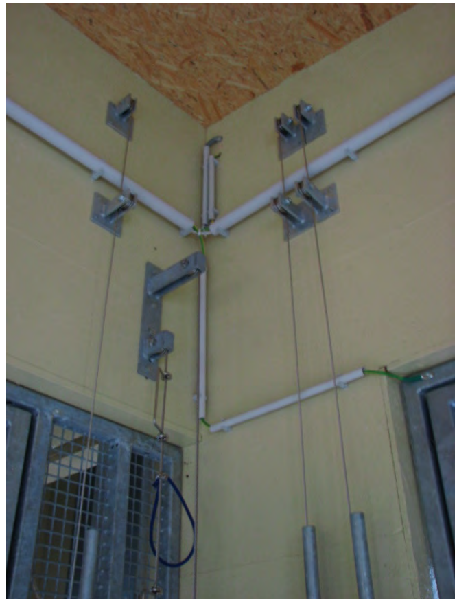
Mechanical gates: All shift doors are operated mechanically which is most reliable and controllable ©Monika Fiby, 2014
