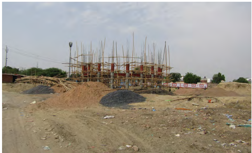
An overhead tank being constructed at the study site. © Mirza Altaf Baig.
