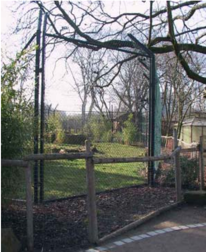
Removable fence panel. The fence panel is removable to allow access into the enclosure. ©Monika Fiby, 2004
