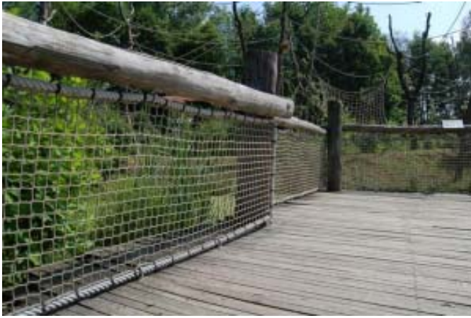
Fig 20. Visitor safety - The nets on the bridge prevent children from falling into the water. ©R.J. van Sluis, 2007
