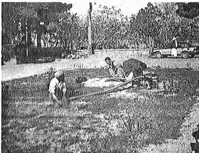
Installation of water pump. Photo by Nick Lindsay.
