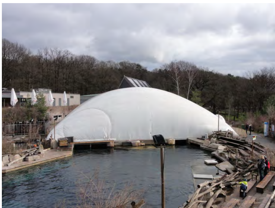
Air dome: During winter, an air dome covers basin 1 and basin 6. ©Jonas Homburg, 2016
