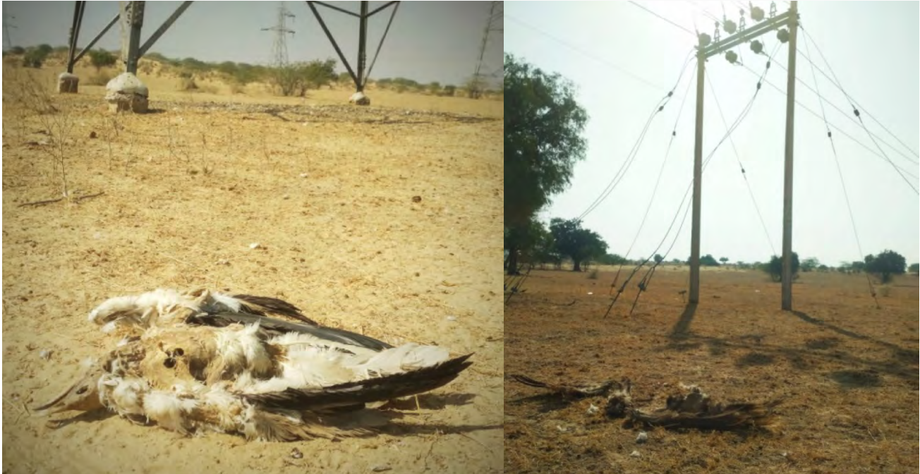
Egyptian Vulture mortality by power lines.
