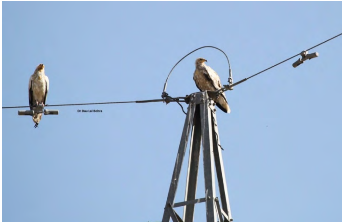
Egyptian Vultures on pylon.
