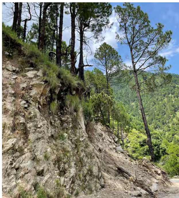
Unmethodically cut hill to broaden roads. The Chir pines stand dangling on the edges. The Chir pine on the extreme right could fall anytime. © Aishwarya S Kumar.
