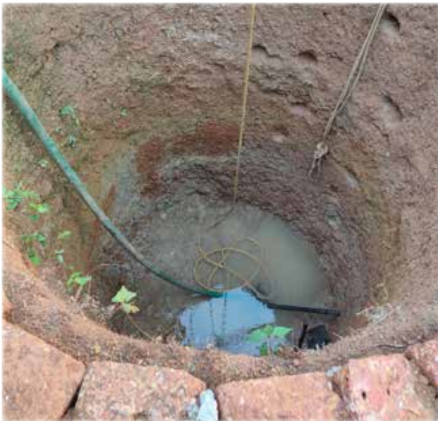
Community members cleaning a laterite well in Chottanikkara, Ernakulam District, to facilitate subterranean fish surveys.
